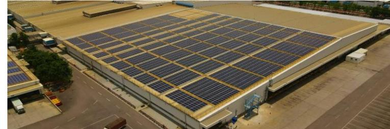
1.6 MW Solar Rooftop on MS Roof
