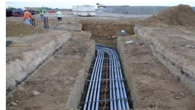
Segregation & digging of Trench in Industrial Area and Underground Cable Laying
